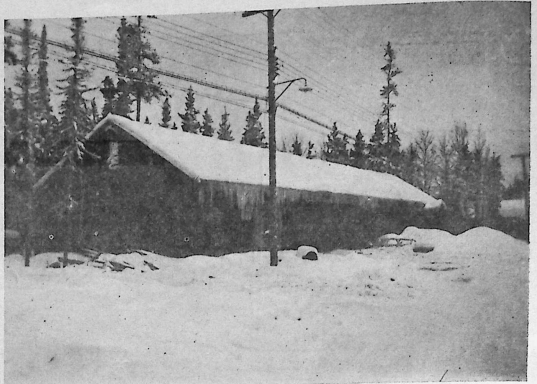
Winter Construction in the Yukon
